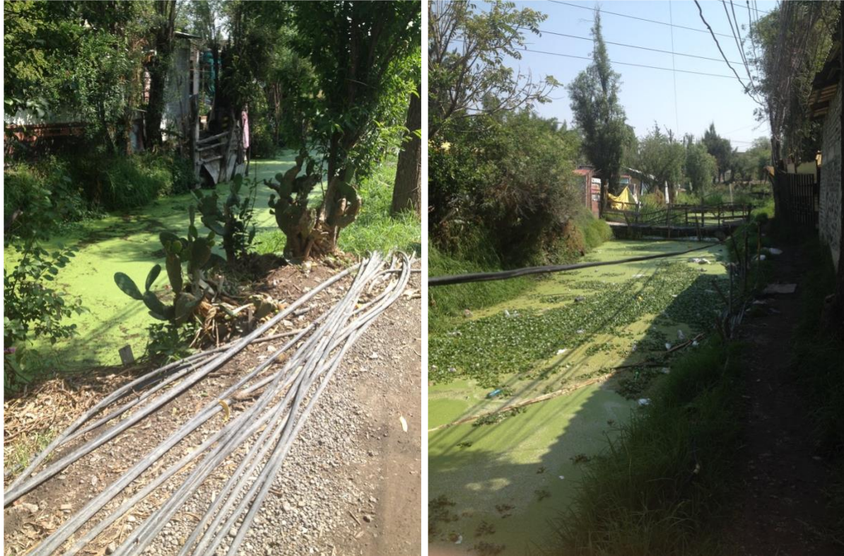
Figure 8.2 Improved water supply in Amalacachico, Mexico City
