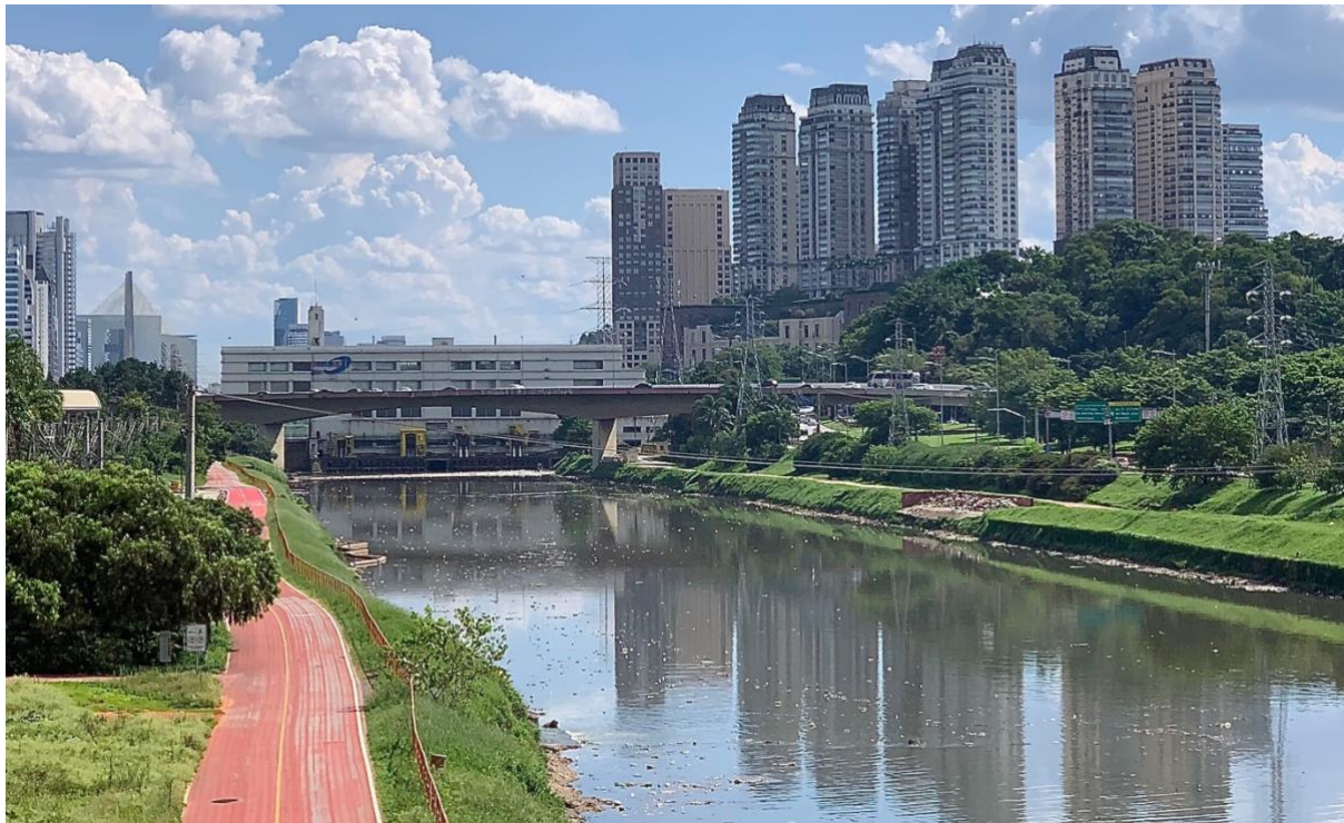
Figure 5.1 Pinheiros River in São Paulo and the Traição pumping station in central São Paulo
